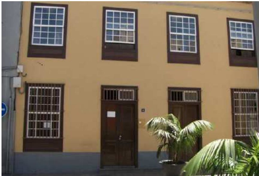
Building of "Obra Social La Milagrosa" C/ Antonio Domínguez Alfonso 5. Nowadays known by Calle de La Noria
